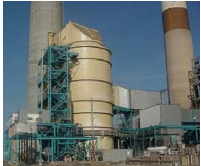
Figure 12a. A Wet FGD Absorber Vessel 7 Figure 12b. Photo of a wet FGD Absorber Vessel 11
